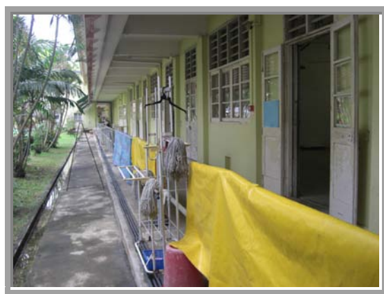
i. Former premises at 29 Jalan Tembusu
